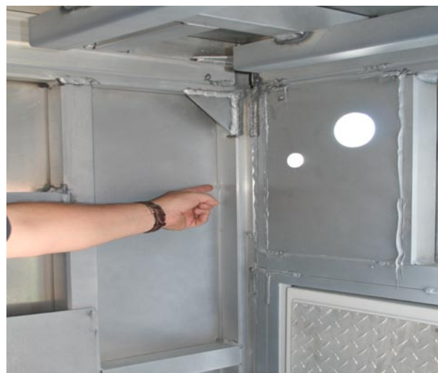
(above) The redesigned full-length adhesive joint is stronger than the earlier skip-welded joint and it excludes moisture, eliminating a source of corrosion.
