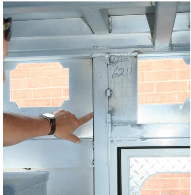
Older body styles used skip-welding to join the aluminum skins and frames. This permitted moisture to penetrate, causing paint and corrosion problems and excessive warranty claims.
